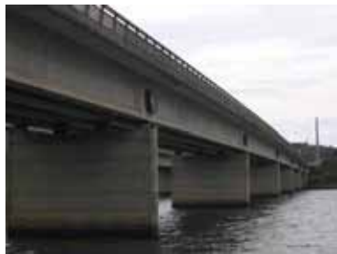
Kings Avenue Bridge piers
