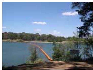
Boom gate upstream of the dam wall
