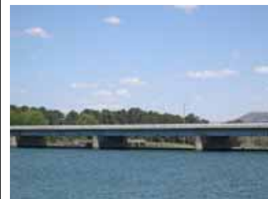
Bridge crossing above dam wall
